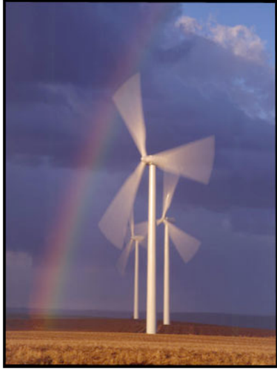
Wind turbine (UC Bureau of Land Management)
