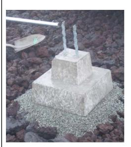
Left photograph shows a placed Pillar block. The block was not well leveled at this time. We need a water level to check the local level of the pea gravel.
