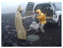
Second, we lifted the pillar block by the pole as tested at UHH. The weather was very bad (it was raining heavily). I think we can place several pillar blocks by ourselves with this method. However, we need crawler crane to place large amount of blocks
