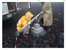
When placing, the pillar block sank a little bit due to the movement of pea gravel. It might be difficult to adjust levels below 1cm, but I think it is possible to adjust the level between blocks within 2cm. As Jay suggested, tamper would be helpful.
