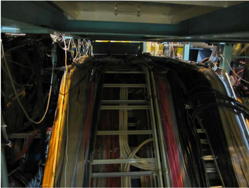
Fig.8 Cables on the top of Belle structure. (Nov.22,2010)
